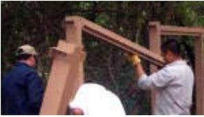
Once the rails are in place concrete the remaining posts in place checking for plumb and continuing down the fence line until all posts are set, plumb and square. It's a good idea to wash off excess concrete splatters on the fence while concrete is still wet. Then, allow an appropriate time for the concrete to set up.
