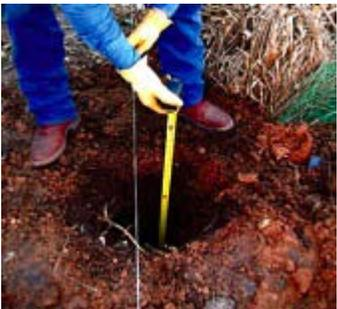
As you drill the holes, place the posts in holes BUT DO NOT cement them in place yet. Start with one corner or end post place the bottom receiver on a 2X4 to regulate the height of the bottom rail to one and one half inches above ground level. Then, making sure that it is plumb (level) and that the attached receivers are facing
