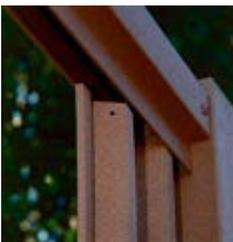
Using steps 1,2, and 3. Repeat this for each picket until the last four to five pickets. Place those pickets into the rails but don't screw them in just yet. Screw into place the picket closest to the opposite end post, aligning it with the post. Spread or contract the remaining four to five pickets to even the spacing and screw them in top and bottom.
