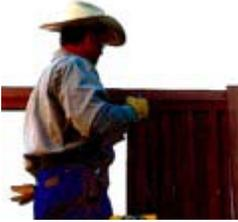
Once you've finished installing all of the pickets on the face side of the fence, move to the opposite side and have a helper install the screws on the back side by pressing a piece of lumber against the overlap of the face side of the picket. Install screws in the short part of each picket at the top and bottom. Continue across the entire panel. At the corner, install a screw in the long side of the last picket and the top and bottom. Place the 4"X4" cap on the post.
